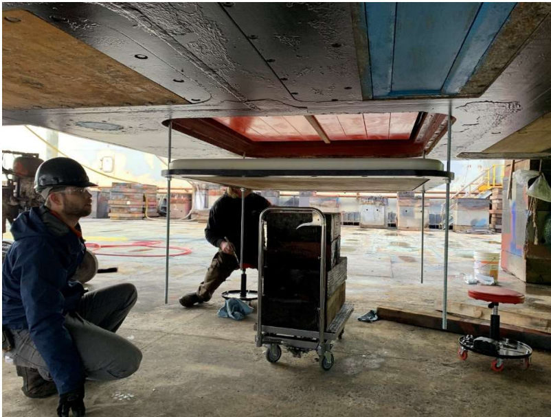
Figure 10.1: Installation of the PS-18 TOPAS array. Photo: E. Roth.
