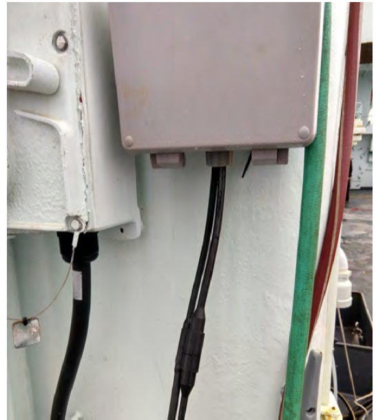
(b) junction box and wet mate connectors
