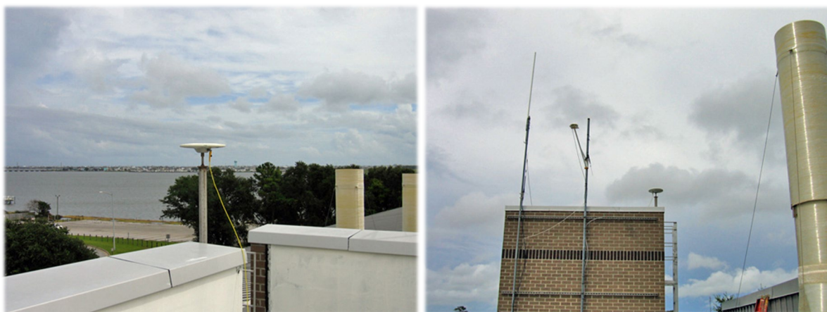
Figure 2. Base station on top of UNC IMS used for broadcasting RTK-GPS corrections to the survey vessel.
