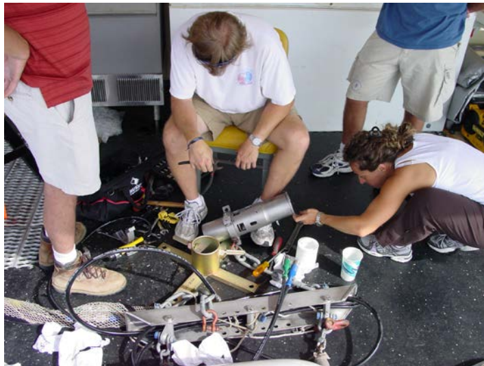
Figure 7. Replacing the o-ring on the airgun.
