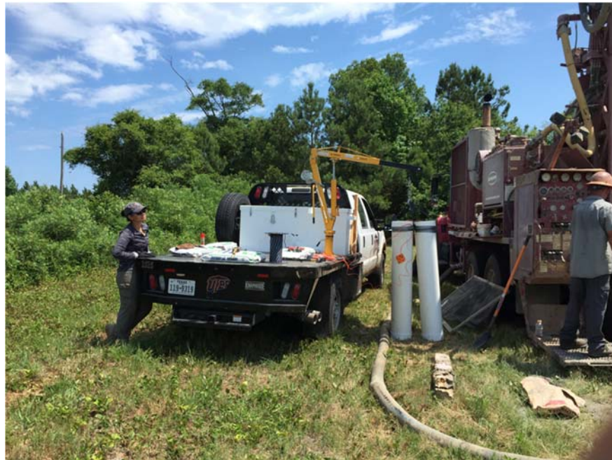
Two charges ready for loading into the borehole. Charges contain 200 lb. each of emulsion and are 5 feet long and 10 inches in diameter.
