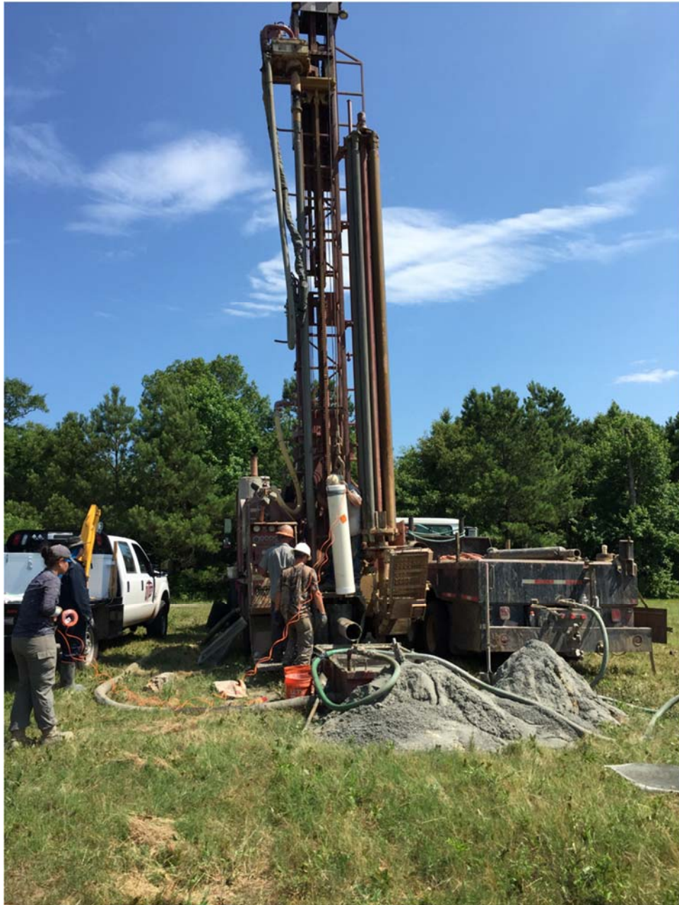
A charge being lifted by the drill before loading into the borehole. Note the two large piles of sand produced from drilling the borehole.
