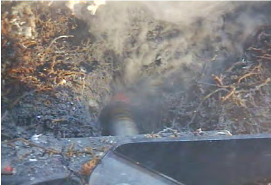
Frame grab #1324: reaming continued, ~3 inch depth of cut
