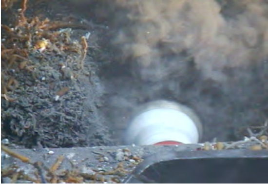
Frame grab #1319: reaming operation, beginning of cut
